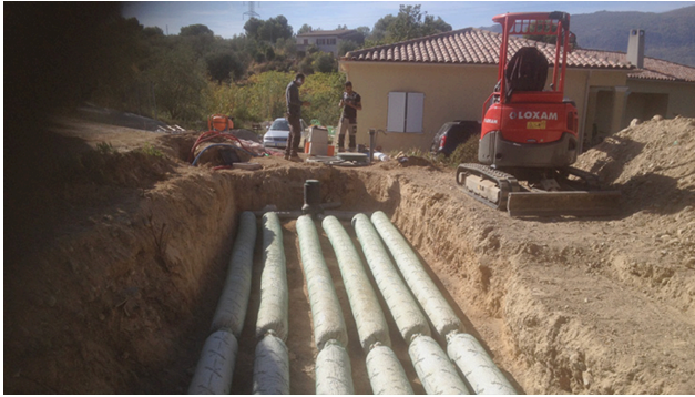
Micro station complemented with drenotube® system - Colomars, France
