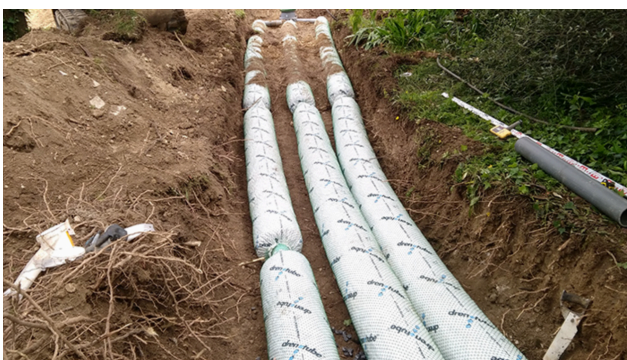
Installation of a compact station followed by drenotube® system - Nice, France
