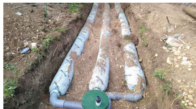
Installation of a compact station followed by drenotube® system - Nice, France
