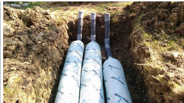
Wastewater treatment plant installed in Opio, France
