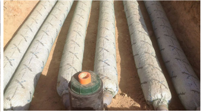
Micro station complemented with drenotube® system - Colomars, France
